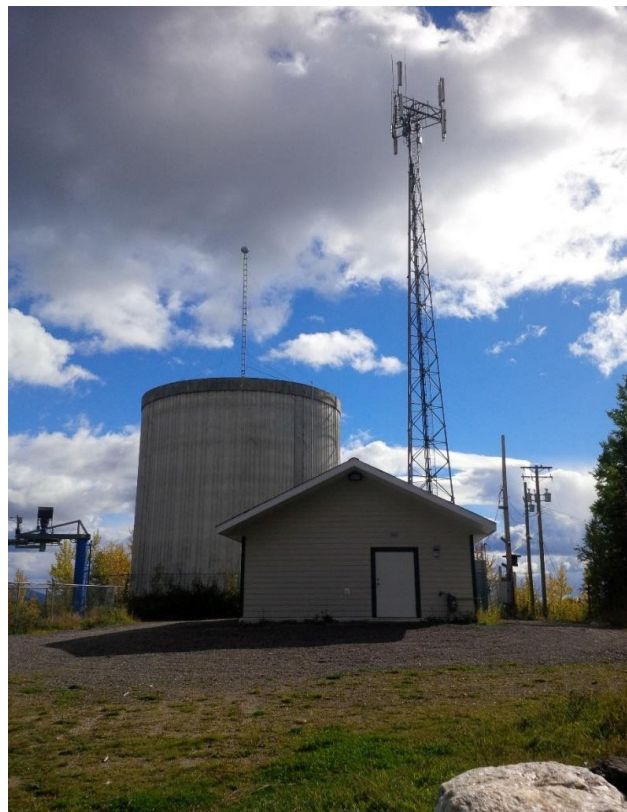
Figure 1: Town Reservoir & Booster Station
