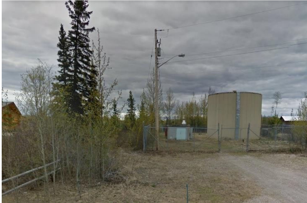
Figure 2: Gantahaz Booster Station and Reservoir
