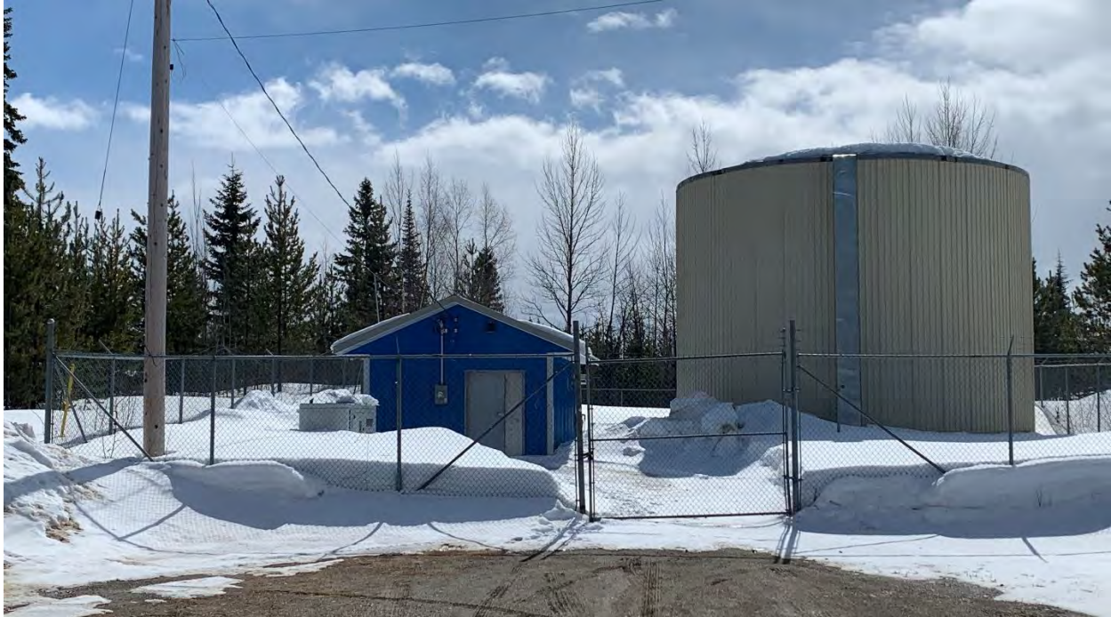
Figure 2.4: Gantahaz Booster Station and Reservoir.
