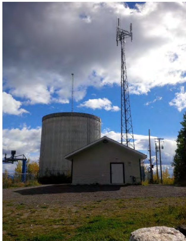
Figure 1: Town Reservoir & Booster Station
