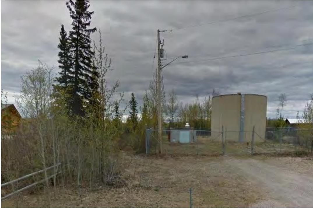
Figure 2: Gantahaz Booster Station and Reservoir
