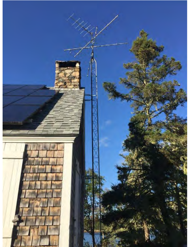
Motus station antennas mounted on a tower bracketed to a building. Photo: Northeast Motus Collaboration
