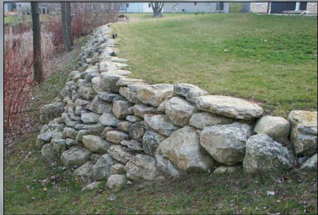
Boulder Retaining Wall
