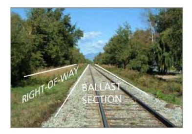
CN will use chemical control techniques on the ballast section and specific locations of the right of way throughout the network for safety reasons. Furthermore, when chemicals are applied via spray train or truck, as outlined in the photo below, additives called surfactants are included to make the chemical work better.
