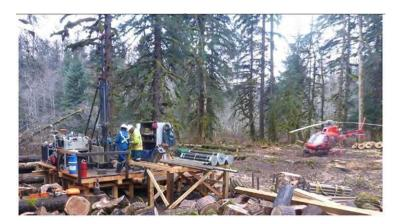
Clearing is required to create a safe workspace at drill pad locations, helicopter landing pads and equipment access trails (this includes deadfall along the edge of a work pad or access trail).
