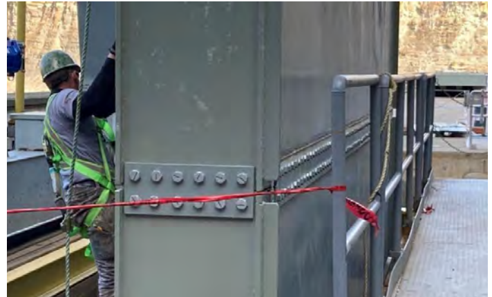
Refurbished PCN draft tube maintenance gate section.
