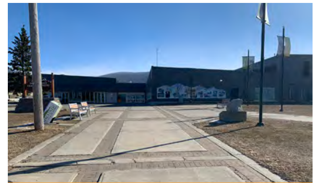
Outside of the Mackenzie Recreation Centre and Library.
