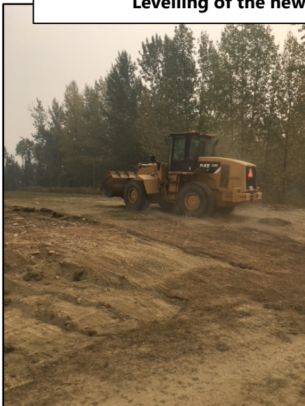
Levelling of the new non-service RV sites
